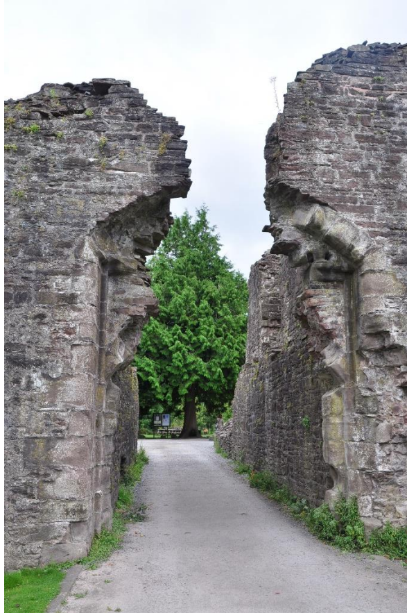
Original castle entrance Gatehouse
